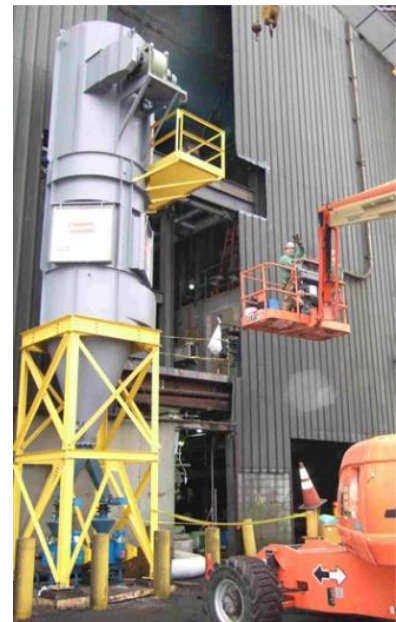
Figure 7. Coal-Sweep Air Separator
